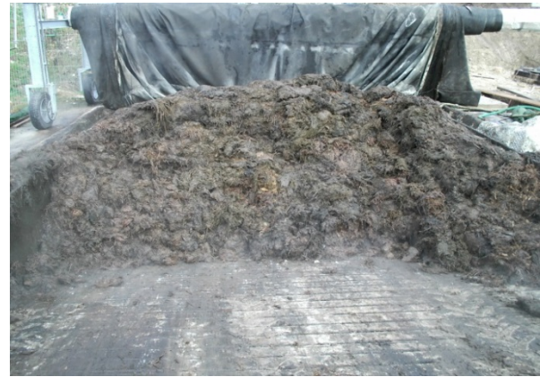
Foto 3: Removal of the old substrate: the poor fermented substrate is separated.
